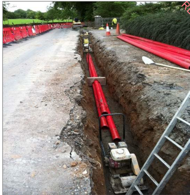
Figure 6 - Typical 38kV Underground Duct Installation
